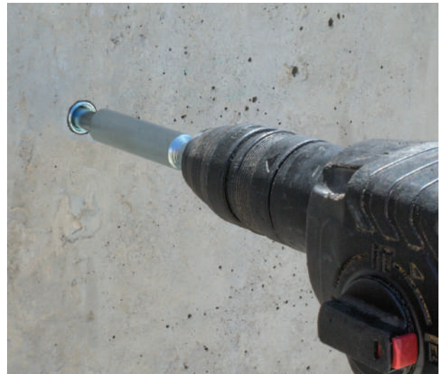
Anchor being set with SDS setting tool.
