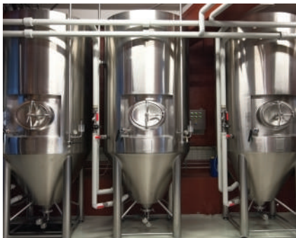
Typical high-corrosive environment — food-processing plants.
