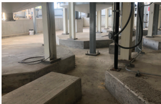
Typical medium-corrosive environment — exterior anchorage.
