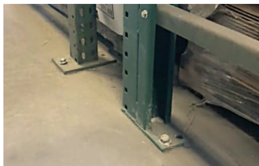
Typical low-corrosive environment — interior warehouse.
