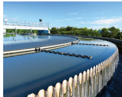
Typical severe-corrosive environment — wastewater treatment plants.
