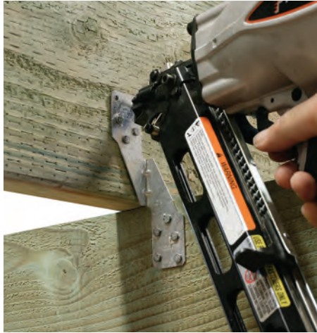
Strong-Drive® SD CONNECTOR Screw
