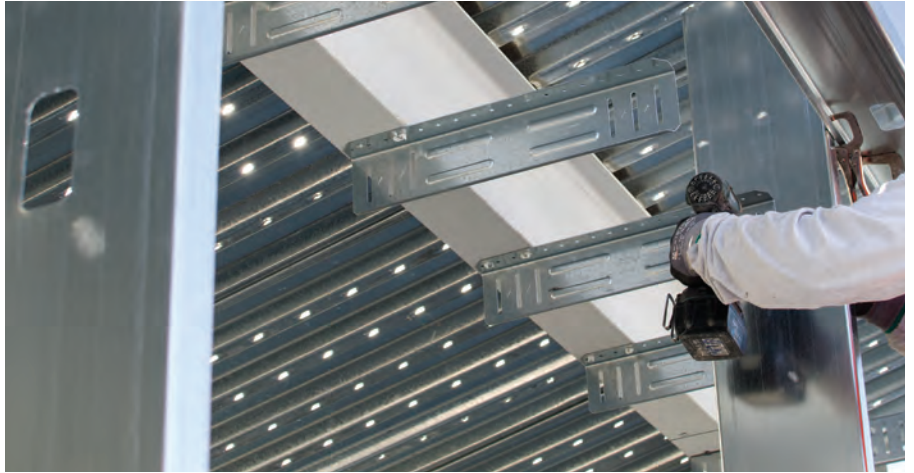
Strong-Drive SDS HEAVY-DUTY CONNECTOR Screw
