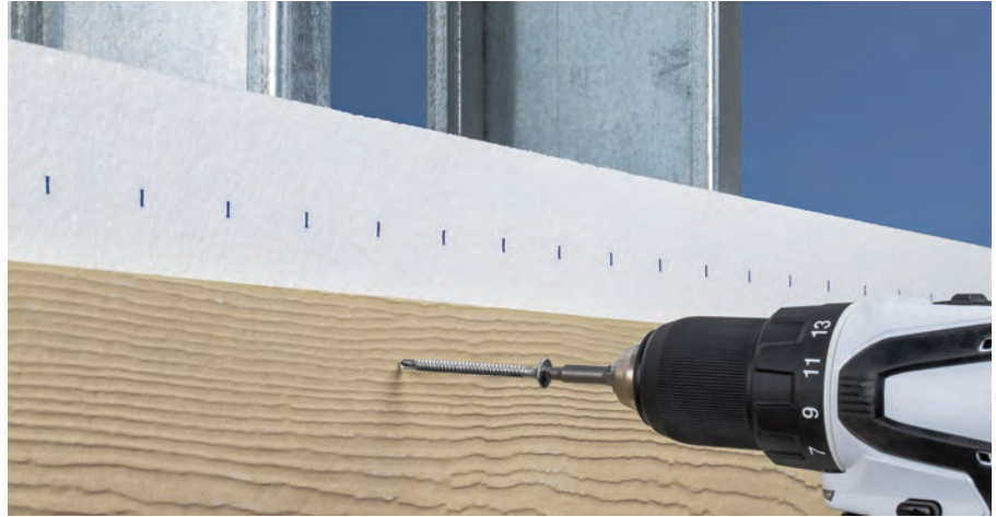
Wire-Lathe Modified Truss-Head Screw
