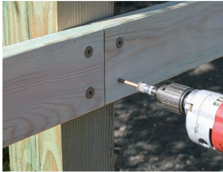
Strong-Drive® SDWS FRAMING Screw
